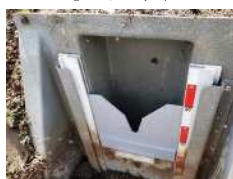
落水柵・流量調整板
